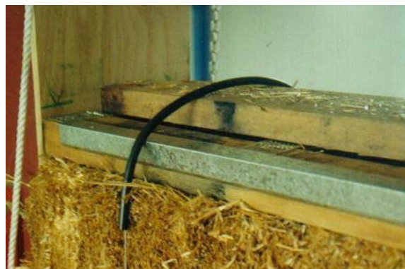
Figure 3: View of top plate assembly showing sleeved wire loop. (Photograph P. Florence)
