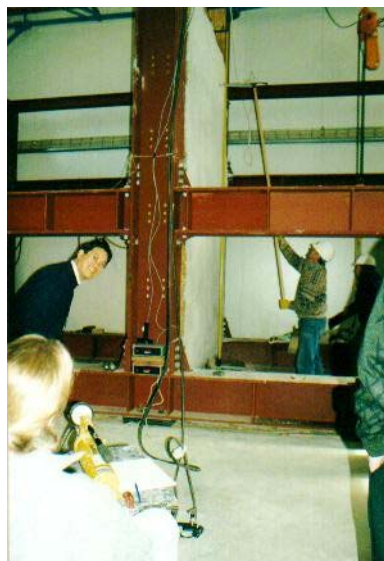
Figure 9: View of lateral measurement process. (Photograph P. Love)
