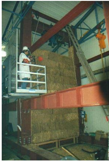
Figure 4: Trimming wall to size. (Photograph P. Florence)
