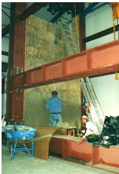
Figure 5: Render application over mesh and straw bales. (Photograph P. Florence)
