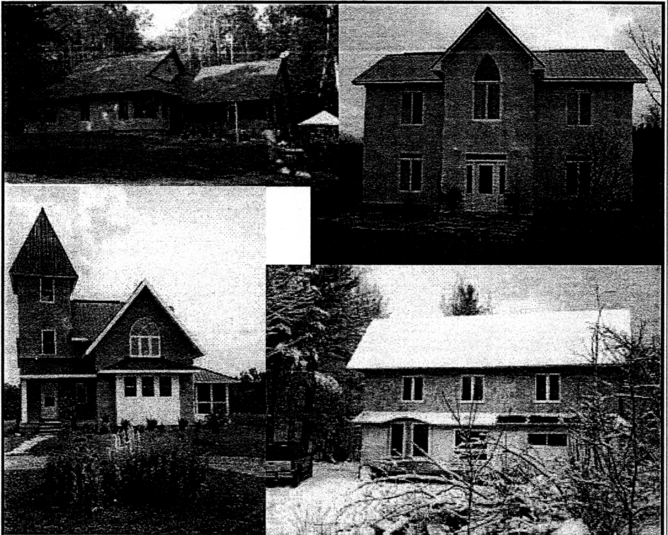
Straw Bale homes in Ontario come in all shapes and sizes. Clockwise from top left: The Smith/Marcotte home, Bancroft; the Cook home, Kanata; the Wise/Jansman home, Centreville; the Beacon/Magwood home, Madoc.
